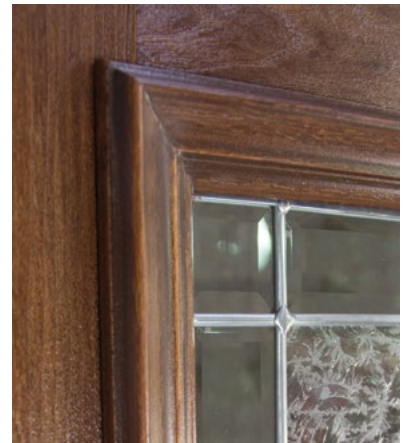
Door moulding shown here does not use unsightly screws to mount the frame to the door.
